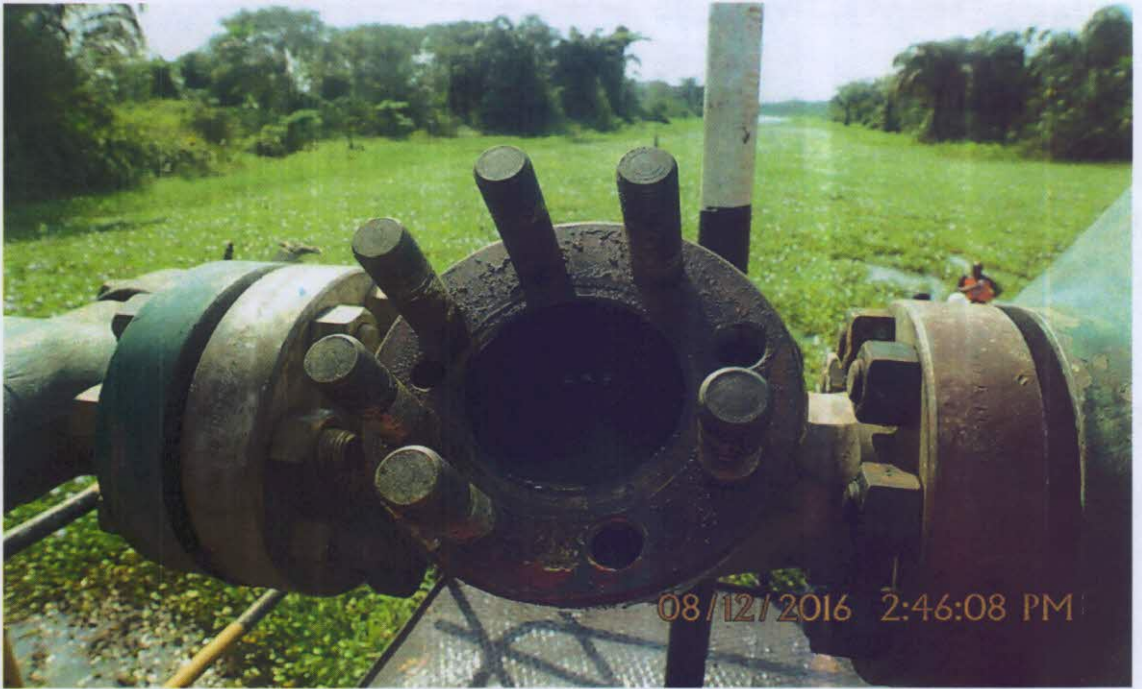
SPILL POINT – SUB-SURFACE SAFETY VALVE (SSV) WAS REMOVED
